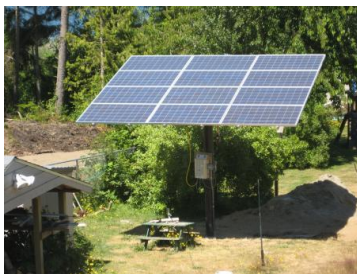
Dual axis solar energy tracking system at the Sawitzki residence in Poulsbo
